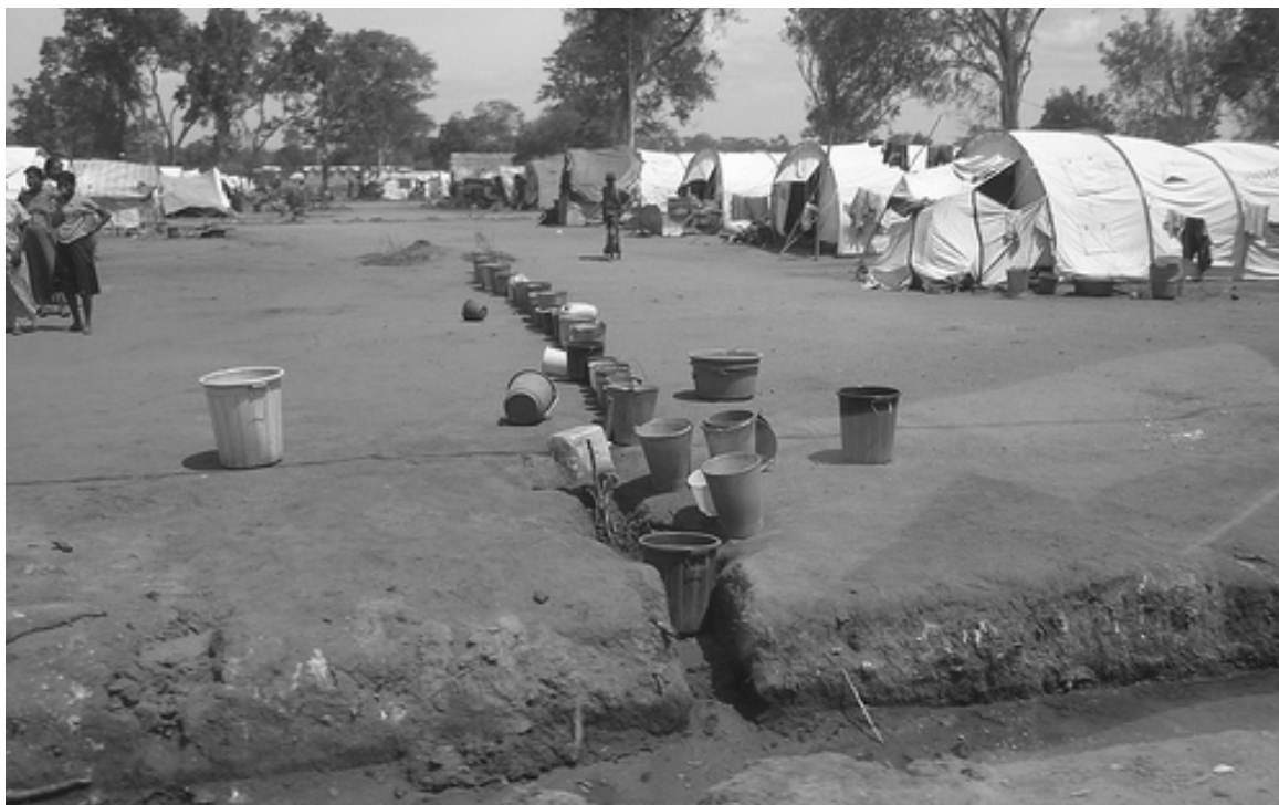
Drainage systems in the camps across Vavuniya have already proved insufficient during 3 days of rain in August. The monsoons are expected to be much worse, but there are no plans to shut down the camps
